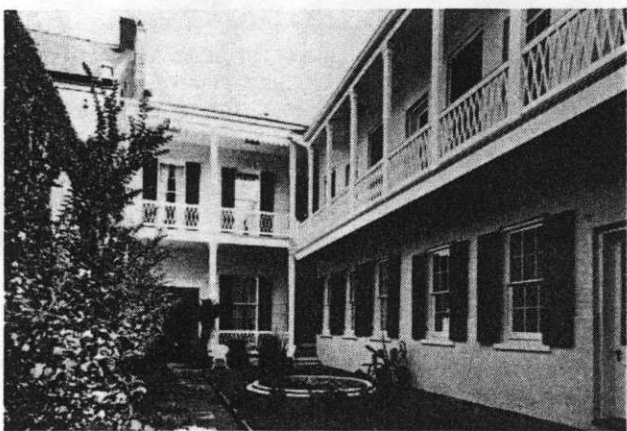
Fig. 4 The rear courtyard and galleries (Photo courtesy of Gallier House)
